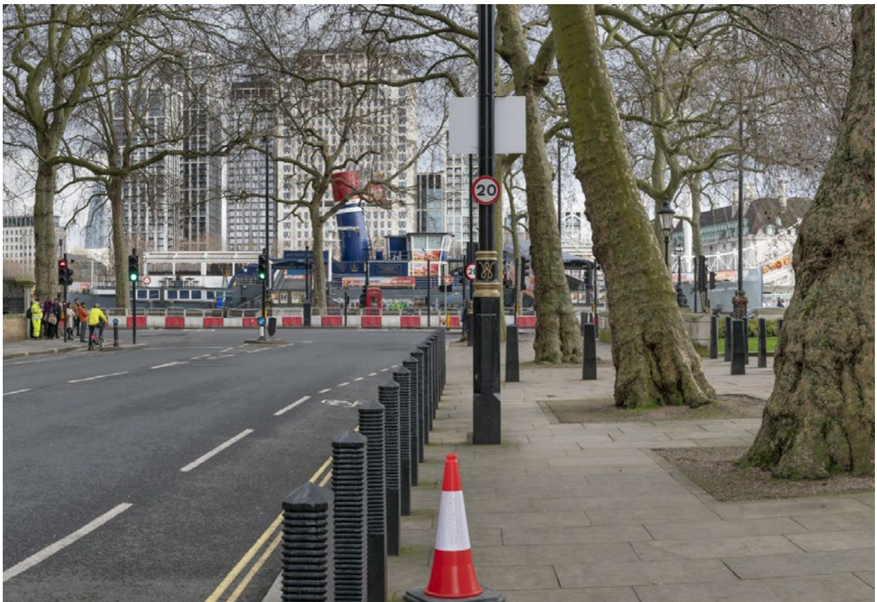
Figure 2.9: View along Horse Guard's Avenue towards the river at high tide - as proposed
