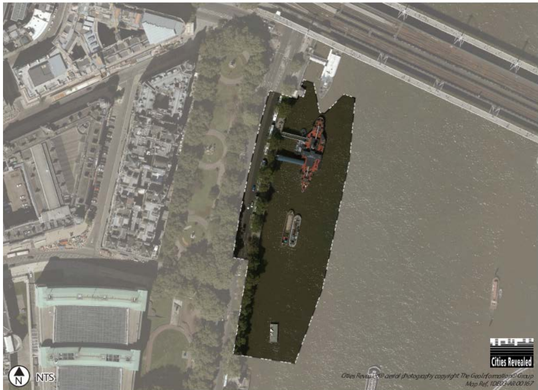
Figure 1 – Site Before Construction Commenced
